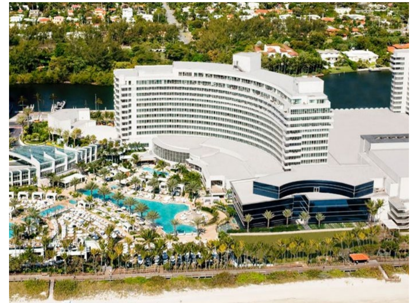
Sorrento Tower at Fontainebleau, Miami Beach, FL
