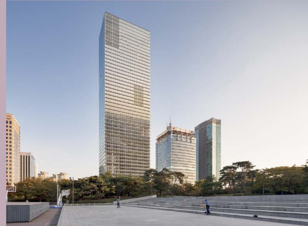
Project: FKI Tower Location: Seoul, South Korea
